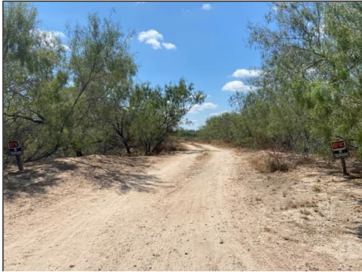
Photograph 60 – View looking south at the culvert crossing located at Private Culvert Crossing 1.
