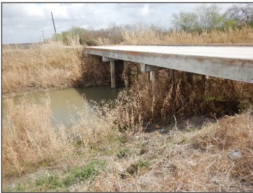
Photograph 38 – View looking north at the concrete bridge located at County Road 205.
