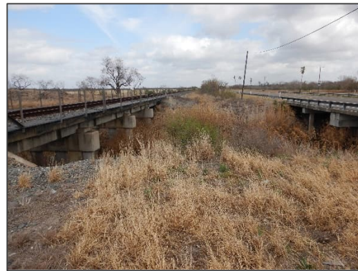
Photograph 41 – View looking north between the railroad crossing and the road bridge located at US Highway 77 Business.
