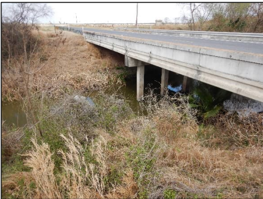
Photograph 15 – View looking northeast at the road bridge located at FM 493.
