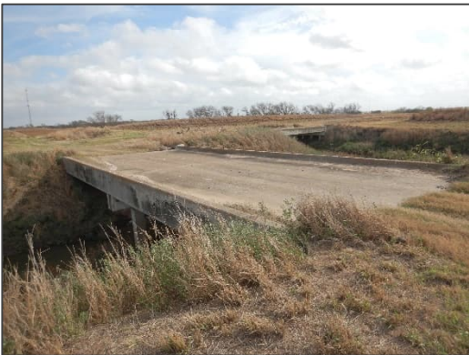
Photograph 21 – View looking northeast at the concrete bridge located at County Road 30.
