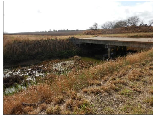
Photograph 22 – View looking southeast at the concrete bridge located at County Road 3000.
