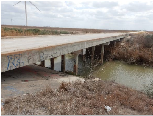
Photograph 49 – View looking southeast at the concrete bridge located at County Road 330.
