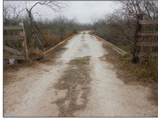
Photograph 58 – View looking northeast at the concrete bridge located at Access Drive 8.
