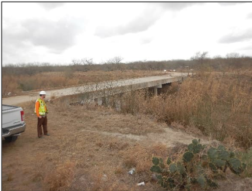
Photograph 32 – View looking southeast at the concrete bridge located at County Road 3600.
