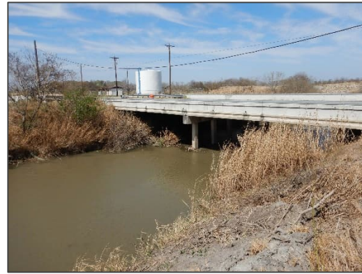
Photograph 28 – View looking northwest at the road bridge located at SH 186.
