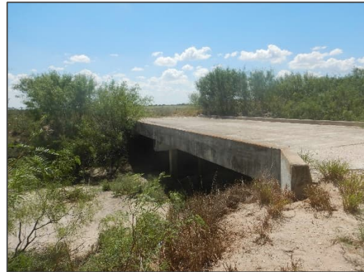
Photograph 17 – View looking southwest at the concrete bridge located at County Road 10.
