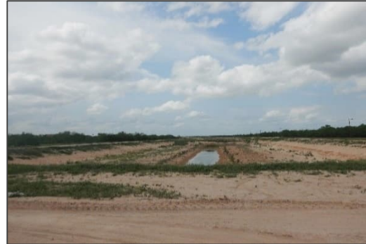
Photograph 4 – View looking north from the culvert crossing located at Cactus Lane.
