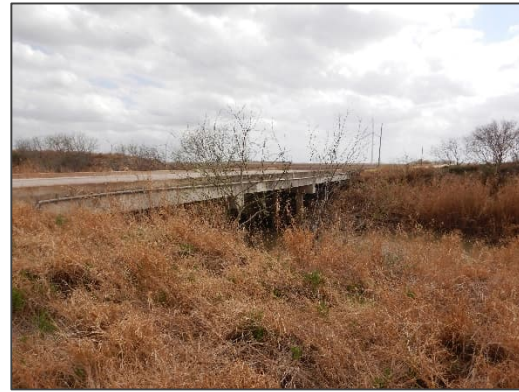
Photograph 52 – View looking southeast at the concrete bridge located at County Road 380.
