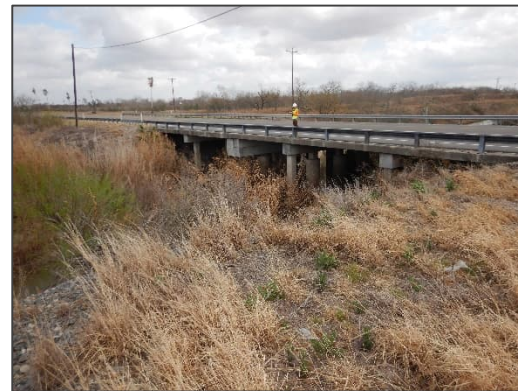
Photograph 42 – View looking northeast at the road bridge located at US Highway 77 Business.
