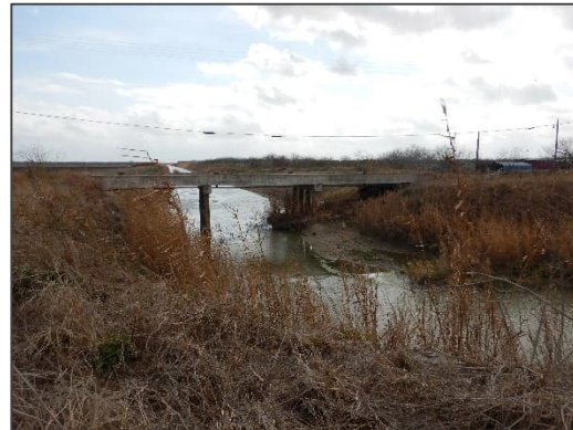
Photograph 35 – View looking east at the concrete bridge located at County Road 156.
