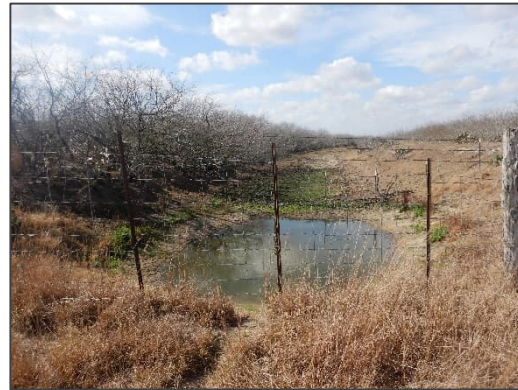
Photograph 10 – View looking south from the culvert crossing located at Unnamed Crossing 2.
