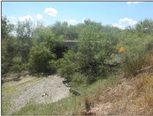
Photograph 13 – View looking southwest at the concrete bridge located at Coolidge Street.
