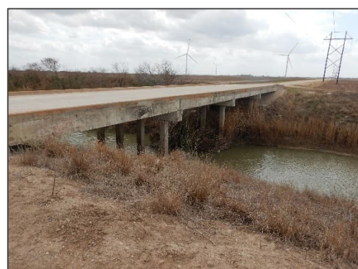
Photograph 48 – View looking south at the concrete bridge located at County Road 315.
