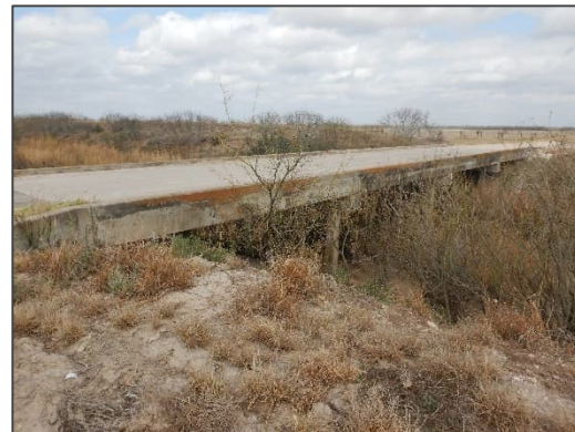
Photograph 47 – View looking northwest at the concrete bridge located at County Road 300.
