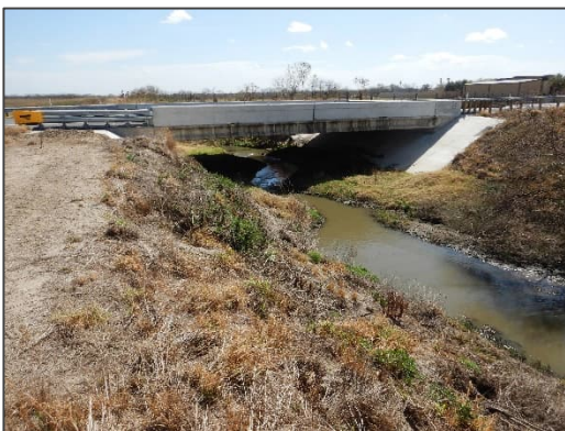
Photograph 27 – View looking east at the road bridge located at FM 1015.
