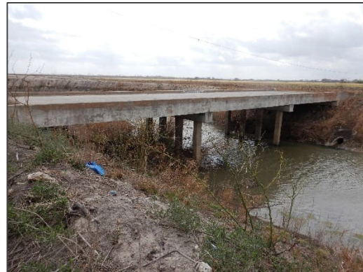
Photograph 36 – View looking northwest at the concrete bridge located at County Road 180.
