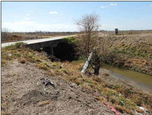
Photograph 26 – View looking southeast at the concrete bridge located at County Road 65.
