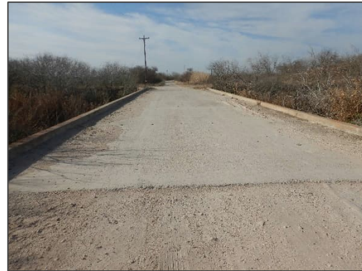
Photograph 30 – View looking northwest at the concrete bridge located at County Road 105.
