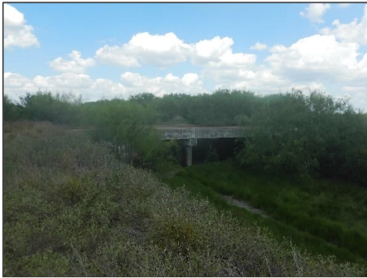
Photograph 19 – View looking northeast at the concrete bridge located at County Road 3000 West.
