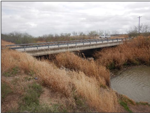
Photograph 72 – View looking northeast at the concrete bridge located at County Road 2900 West.
