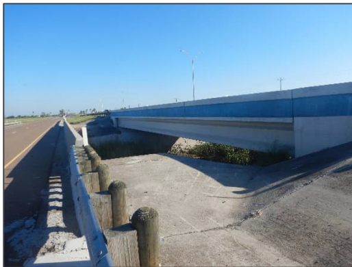
Photograph 44 – View looking northeast at the highway bridge located at US Highway 77 (southbound).
