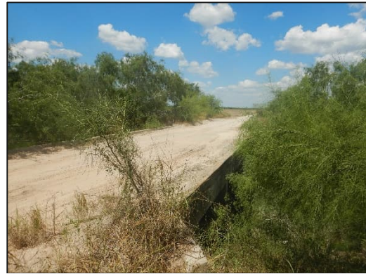
Photograph 16 – View looking northwest at the concrete bridge located at County Road 5.
