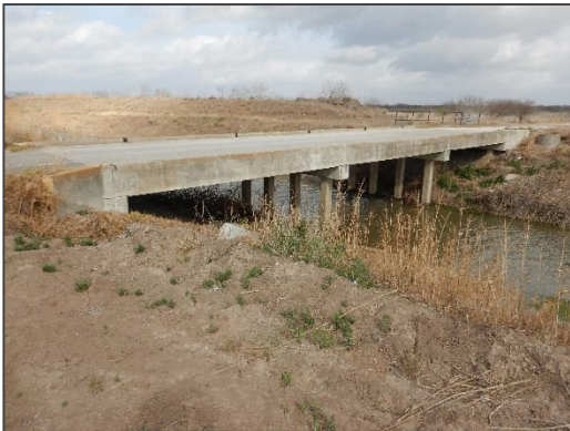
Photograph 33 – View looking northwest at the concrete bridge located at County Road 141.
