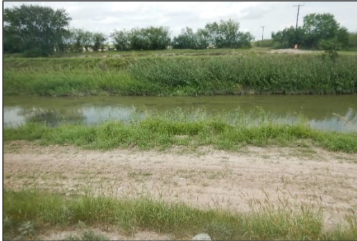
Photograph 1 – View looking south at the location of the proposed control structure which would be situated at the beginning of the project.
