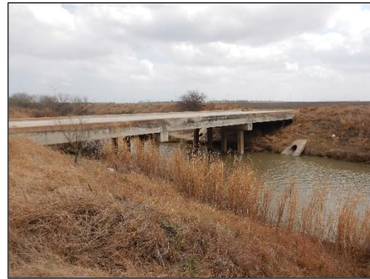
Photograph 54 – View looking southeast at the concrete bridge located at FM 3142.
