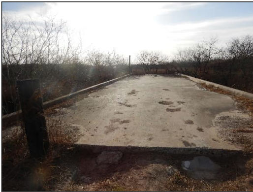
Photograph 31 – View looking west at the concrete bridge located at Unnamed Crossing 4.
