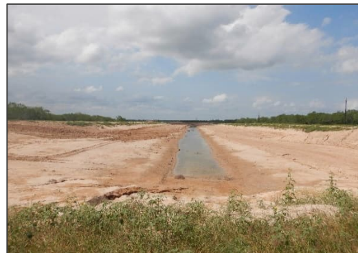
Photograph 5 – View looking north from the culvert crossing located at Unnamed Crossing 1.
