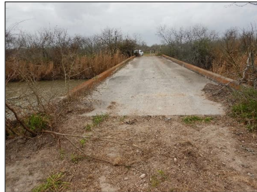
Photograph 59 – View looking northeast at the concrete bridge located at Access Drive 9.
