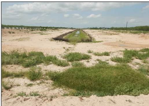
Photograph 2 – View looking north from the proposed control structure located at the begin project terminus.
