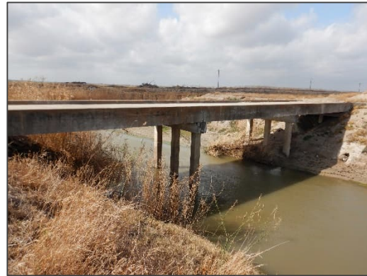
Photograph 34 – View looking southwest at the concrete bridge located at Access Drive 2.
