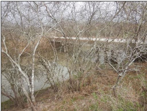
Photograph 57 – View looking north at the concrete bridge located at Access Drive 8.
