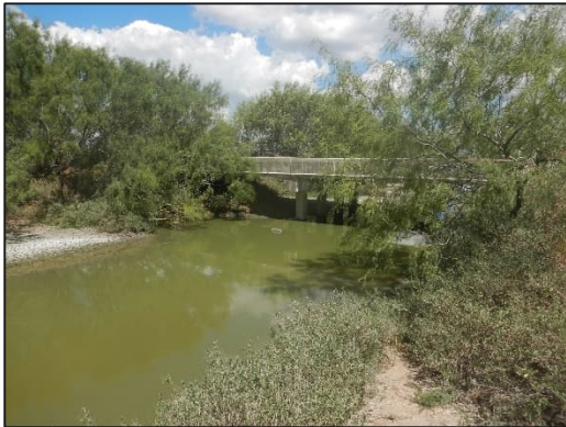
Photograph 14 – View looking northeast at the concrete bridge located at Bucy Road.
