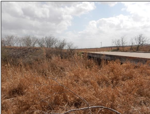
Photograph 56 – View looking southwest at the concrete bridge located at County Road 445.
