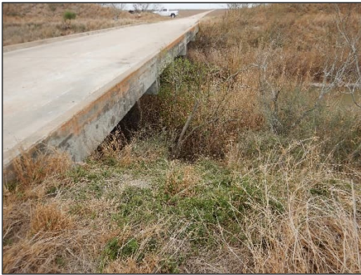
Photograph 50 – View looking north at the concrete bridge located at County Road 345.
