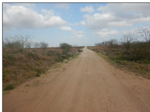
Photograph 65 – View looking east at the culvert crossing located at Mile 25 North Road.
