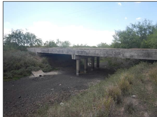
Photograph 18 – View looking southwest at the concrete bridge located at County Road 15.
