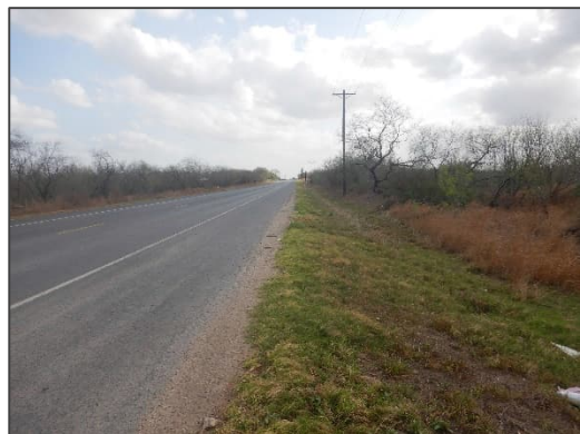
Photograph 64 – View looking south at the road bridge located at FM 493.
