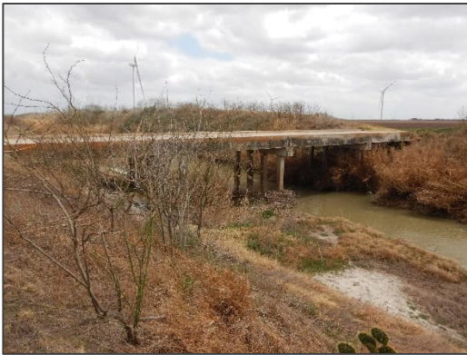
Photograph 51 – View looking southeast at the concrete bridge located at County Road 360.
