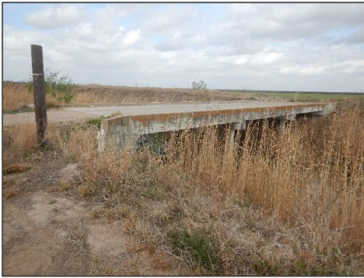
Photograph 37 – View looking northwest at the concrete bridge located at County Road 200.
