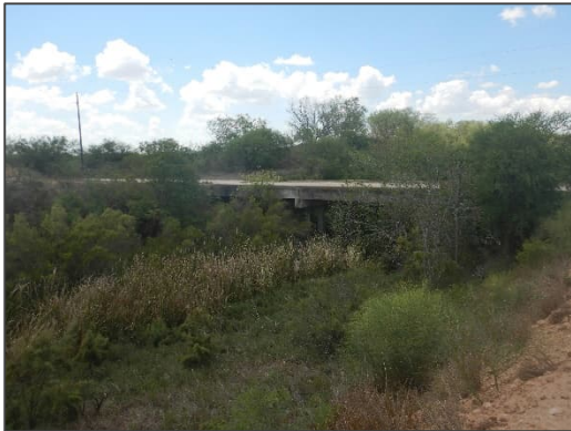
Photograph 20 – View looking southwest at the concrete bridge located at County Road 25.
