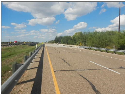
Photograph 9 – View looking north at the highway crossing located at US Highway 281 (northbound frontage road).
