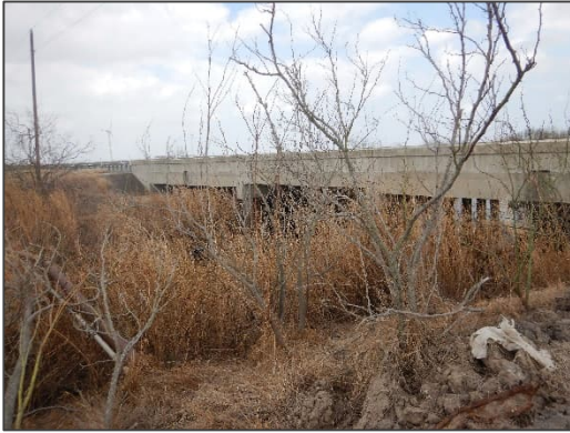
Photograph 55– View looking northeast at the concrete bridge located at FM 2209.
