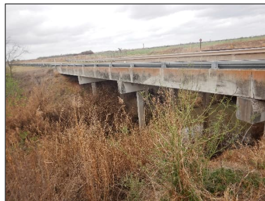
Photograph 71 – View looking north at the road bridge located at FM 490.
