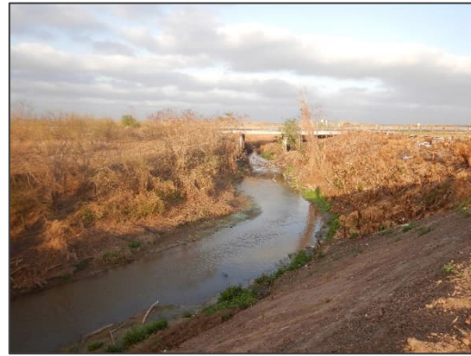
Photograph 69 – View looking east at the road bridge located at FM 88.
