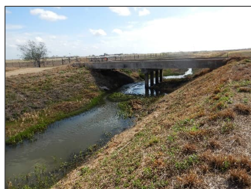
Photograph 24 – View looking east at the concrete bridge located at County Road 40.
