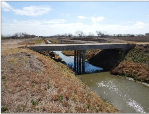
Photograph 25 – View looking east at the concrete bridge located at County Road 60.
