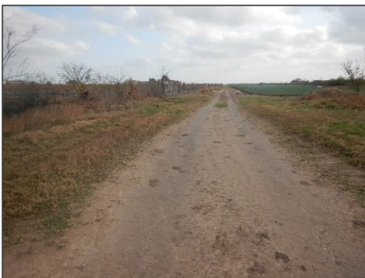
Photograph 68 – View looking south at the culvert crossing located at Mile 5½ West Road.
