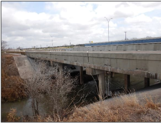
Photograph 43 – View looking northeast at the highway bridge located at US Highway 77 (southbound frontage road).
