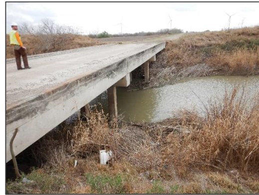
Photograph 53 – View looking south at the concrete bridge located at County Road 398.
