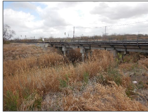
Photograph 40 – View looking northeast at the railroad crossing located parallel to US Highway 77 Business.
